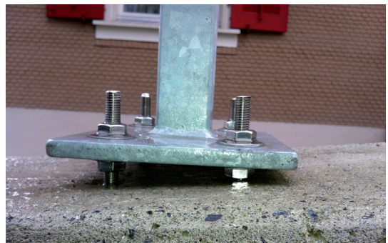
Figure 4: Column fixing with stand-off fixture
