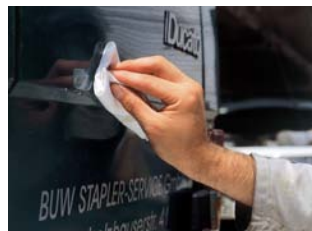
7. Remove remaining adhesive residue using pre-cleaner.
