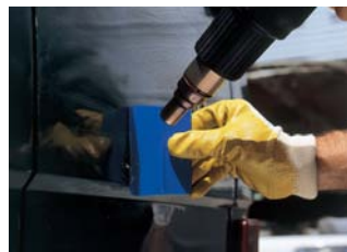
6. Heat up the adhesive residue and remove it using special spatula.
